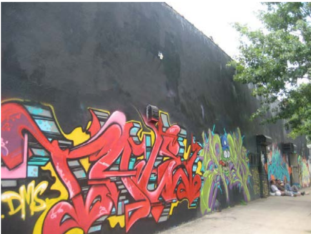
3. View of the north side of the subject property building along East 146th Street.
