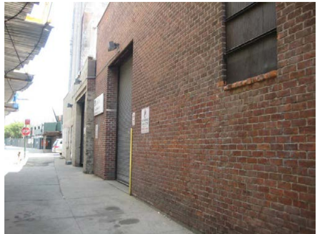
20. View of the adjacent site to the west along Exterior Street/Major Deegan Expressway.
