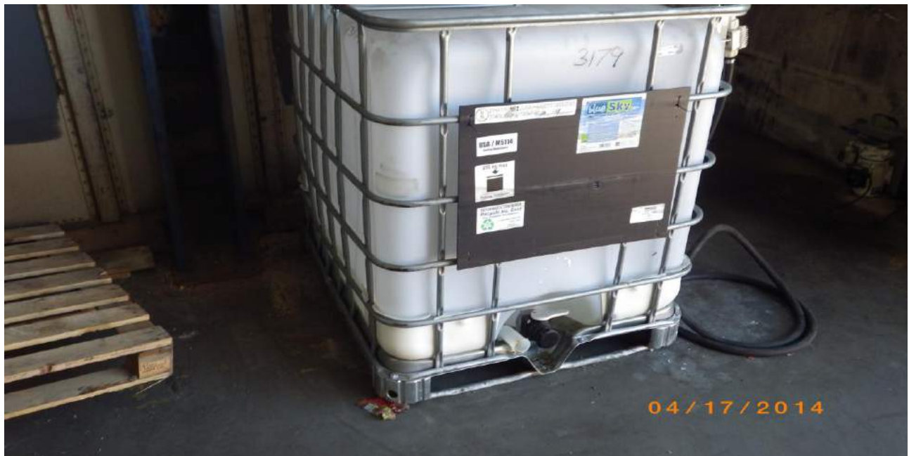
Photo 48: View of the 275-gallon diesel exhaust fluid AST located with the Third Avenue Transit Inc. warehouse.
