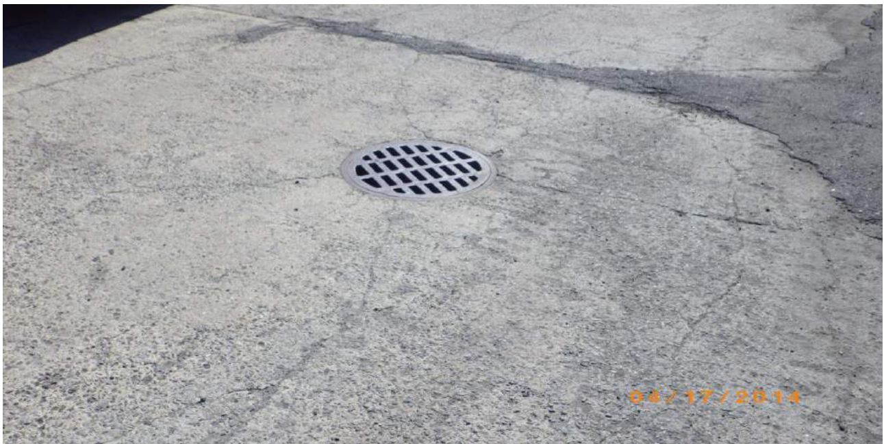
Photo 20: View of parking area storm drain.
