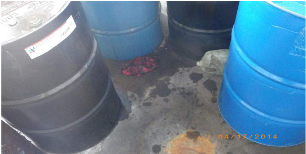
Photo 47: View of recent signs of surficial staining associated with fluid spills.
