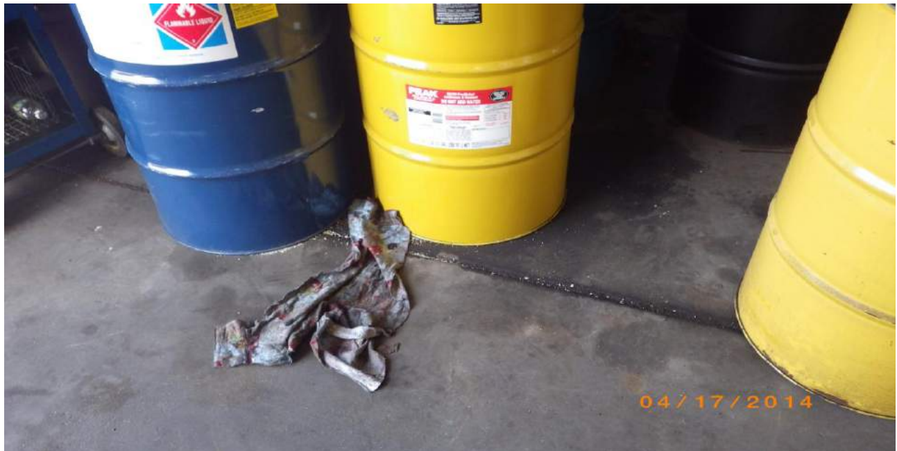
Photo 46: View of recent signs of surficial staining associated with fluid spills.
