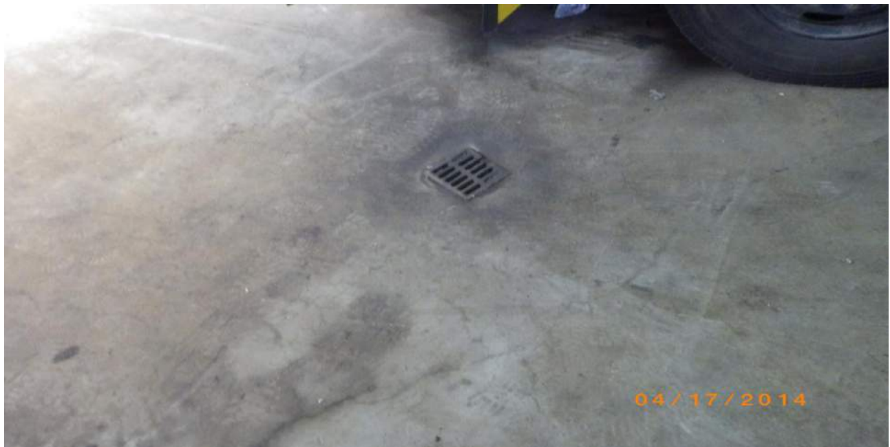
Photo 50: View of floor drain.
