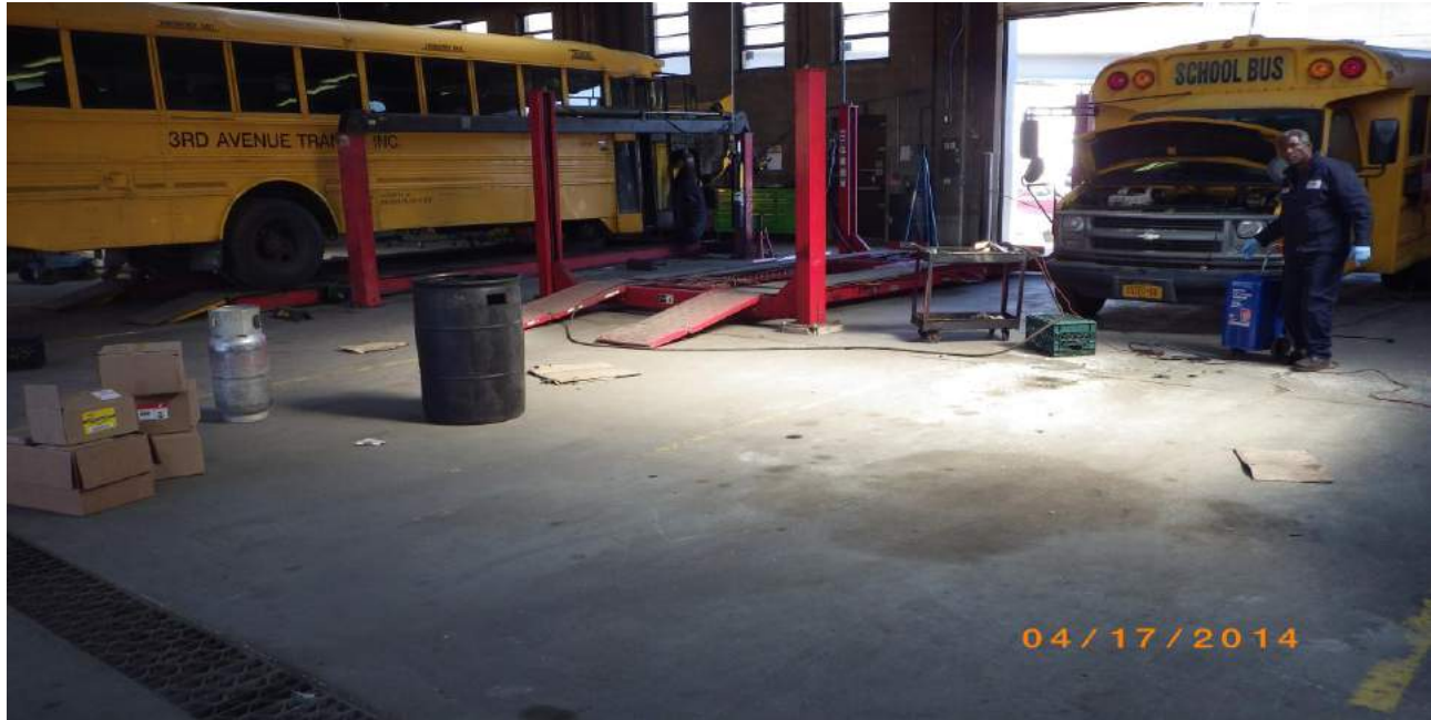
Photo 41: View of the two hydraulic lifts located with the Third Avenue Transit Inc. warehouse.
