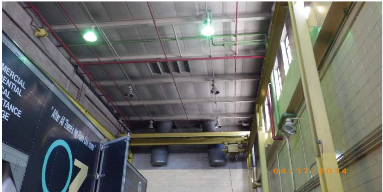
Photo 34: View of the ceiling of the Oz Moving & Storage warehouse.
