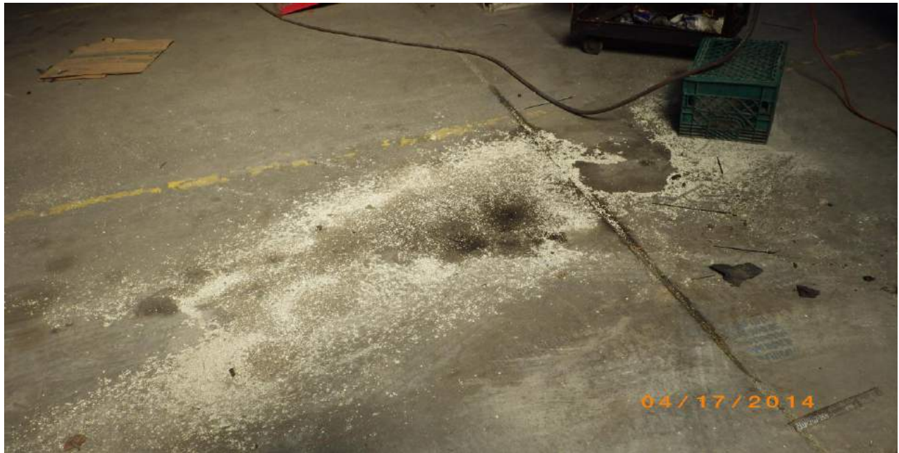
Photo 49: View of recently applied absorbent material located within the Third Avenue Transit Inc. warehouse.
