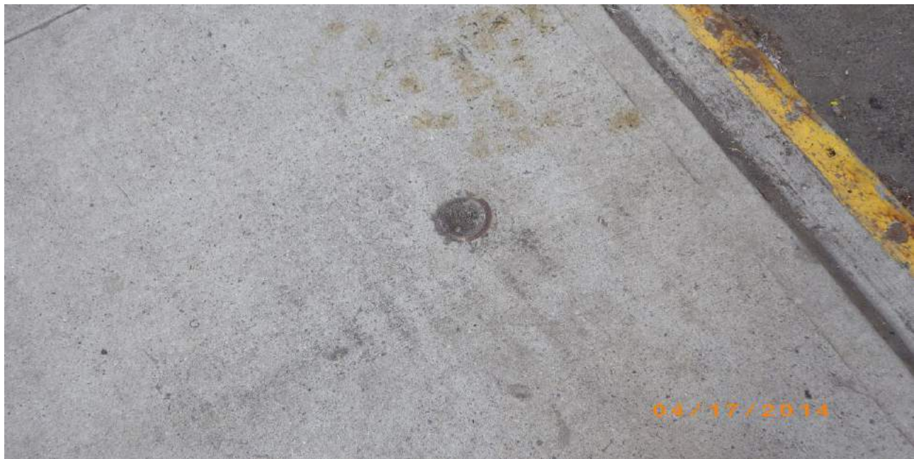
Photo 6: Close-up of apparent fill port.
