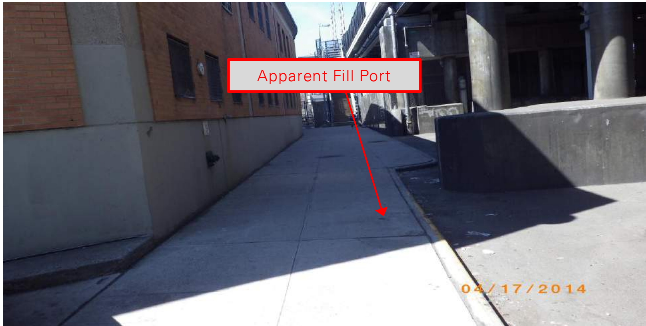
Photo 5: View of the western edge of the Site (facing south). Apparent fill port seen in photo.
