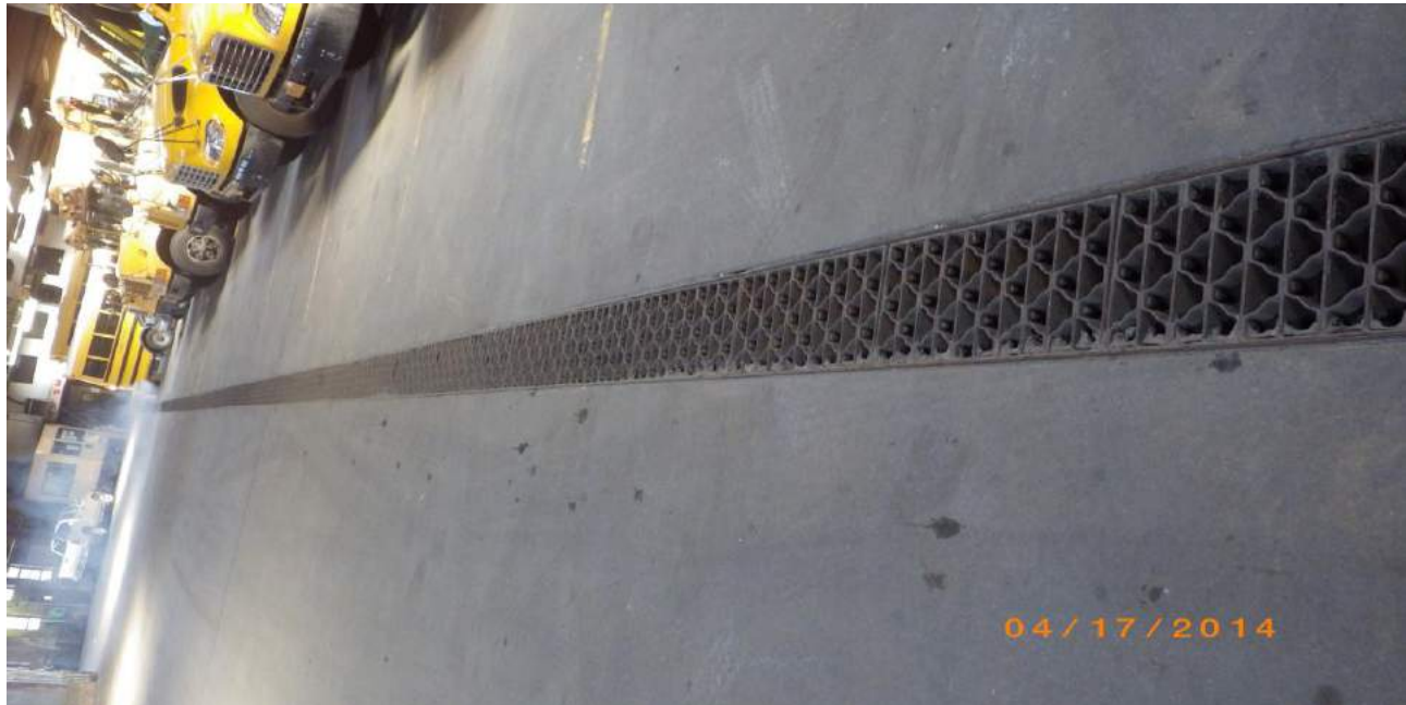
Photo 42: View of the runoff channel floor drain.
