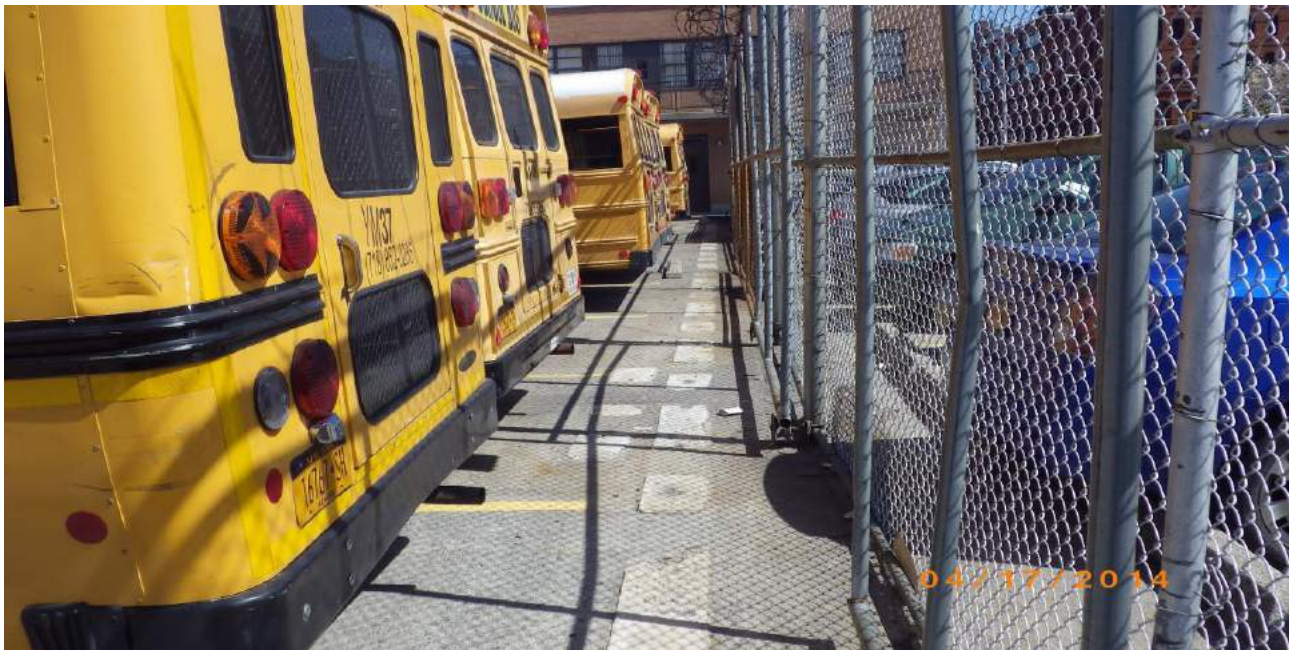
Photo 22: View of the apparent former vent pipes associated with the closed-in-placed USTs.
