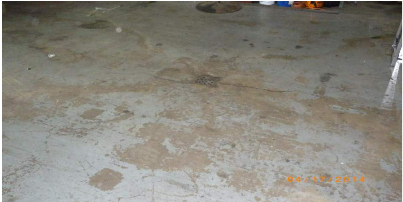
Photo 31: View of floor drain.
