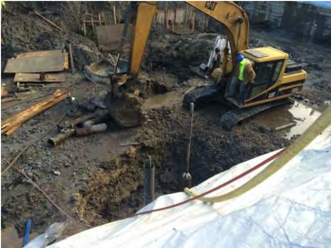
Photo 3 – Additional view of the excavation area, facing east.
